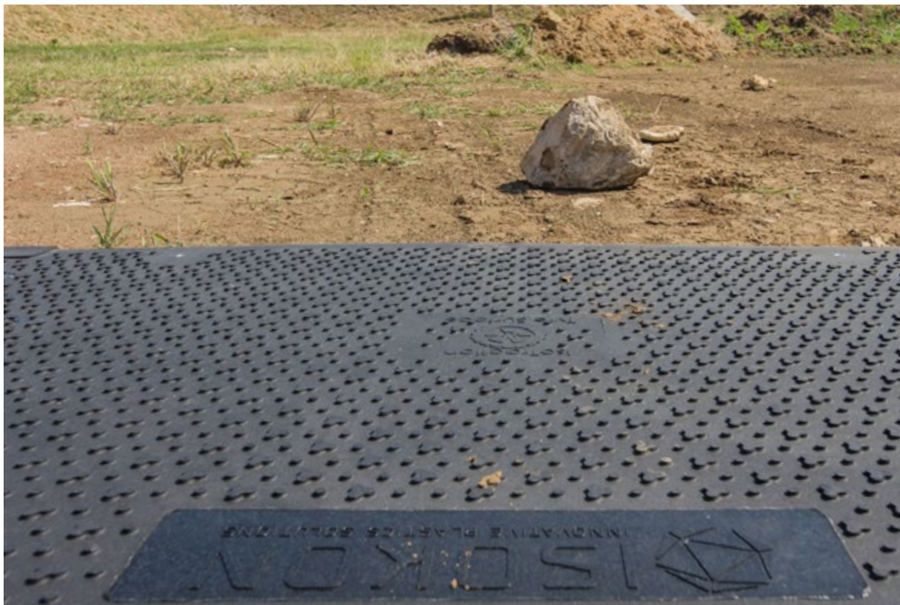
Large boulders or other obstructions should be cleared away.
