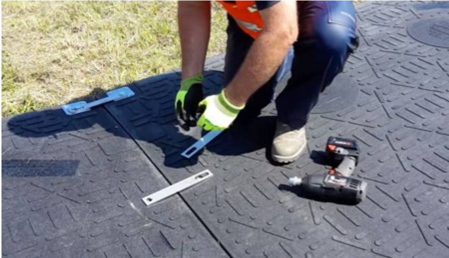
The steel connector strap is aligned over the connection points
