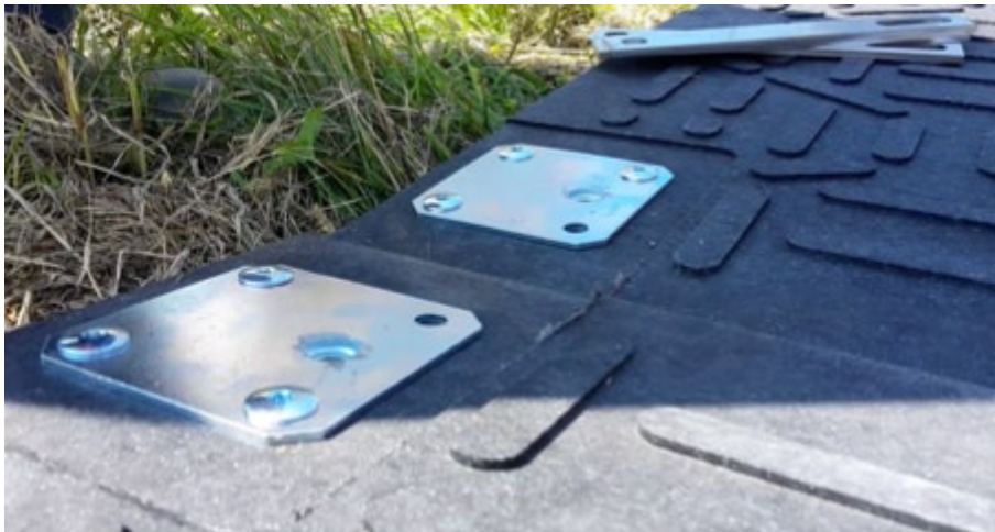
1. Adjacent mats installed ready for connection.
