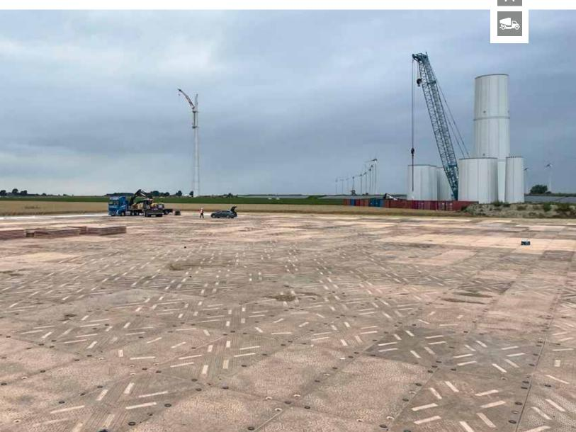
Engineered for performance and strength, the interlocking overlap mats distribute weight across a large surface area while remaining stable and strong through all operating conditions. The IsotractionTM surface tread improves traction and safety for load-bearing vehicles, while the patented Four3 connection system reduces mat drift and slippage. The mats provide years of reusable performance with proper use and maintenance.
